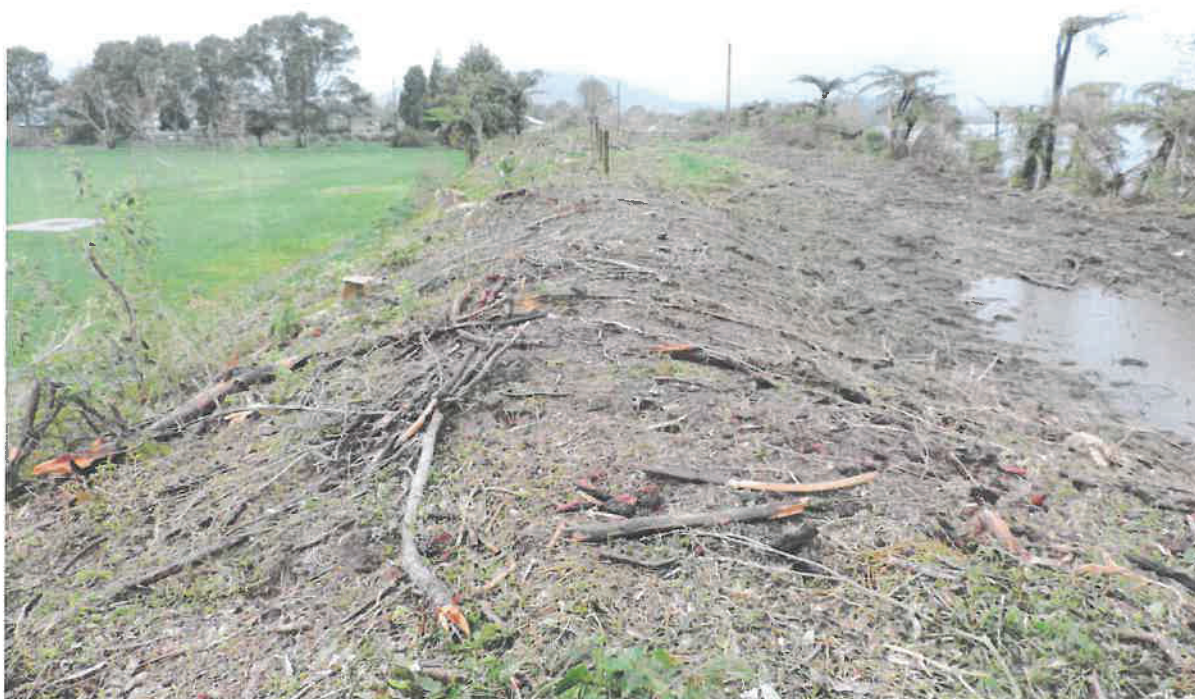
Trees cleared from bank, August 2014
